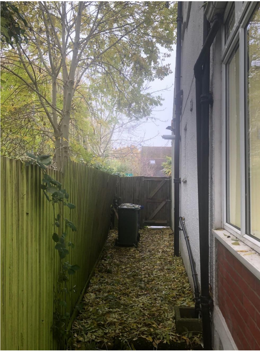
Gap along eastern flank from eastern boundary
